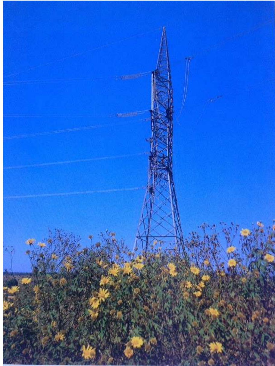
LINEA 220KV, KOLVESI-LUBUMBASHI
