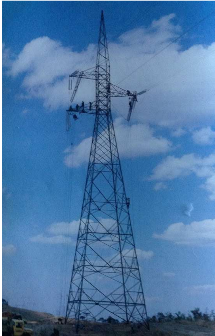
LINEA 220KV, KOLVESI LUBUMBASHI
